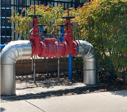
Insulation shall be jacketed finish.
