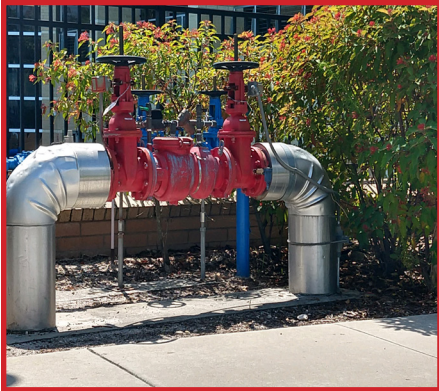
Insulation shall be jacketed finish.
