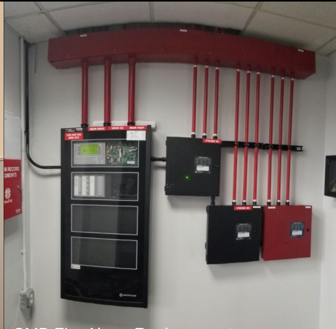
CMB Fire Alarm Replacement
