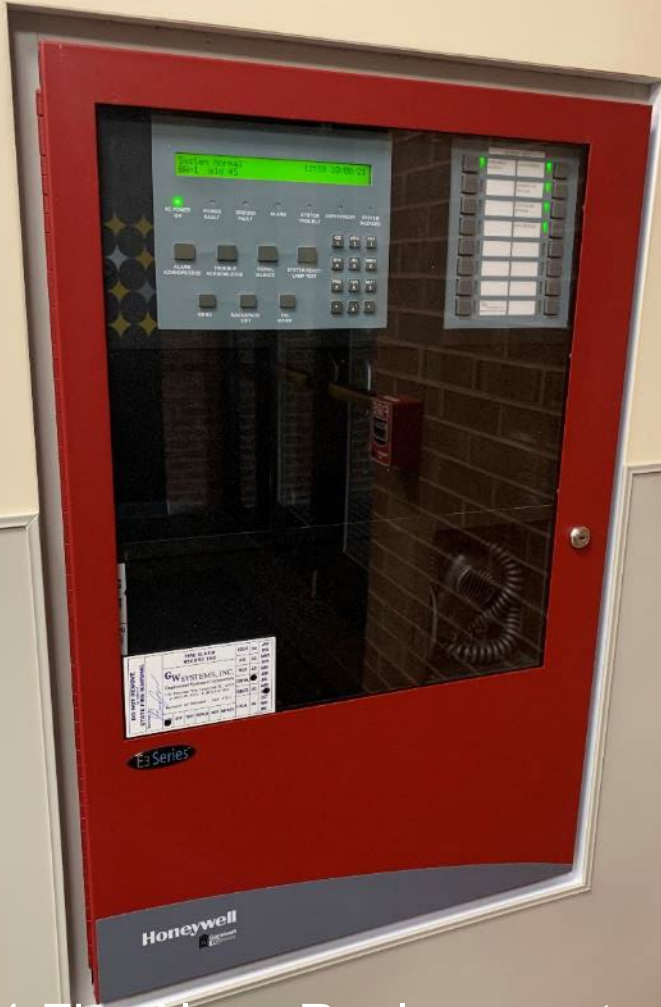
BA1 Fire Alarm Replacement
