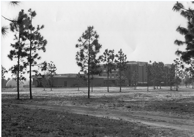
Chemistry Building and Science Auditorium (Theater Building) January 1967
