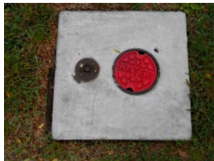
Fire Valve Box with ID
