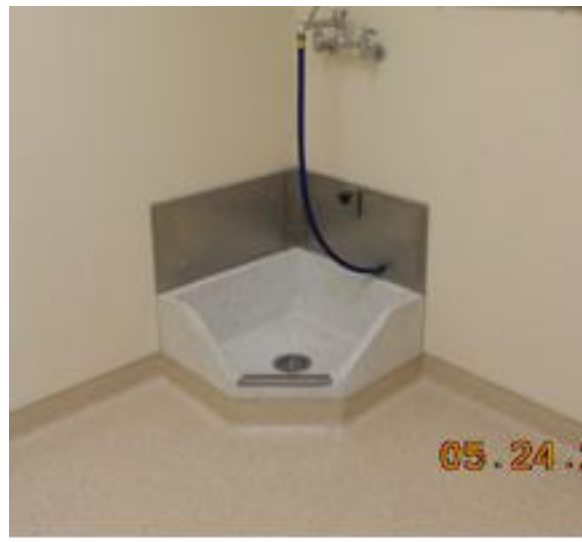
Custodial Room Mop Sink Arrangement
