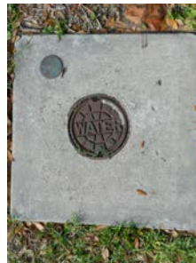
Potable Valve Box with ID
