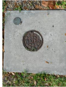
Potable Valve Box with ID
