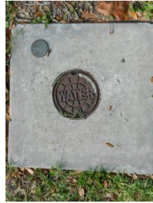
Potable Valve Box with ID
