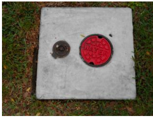
Fire Valve Box with ID
