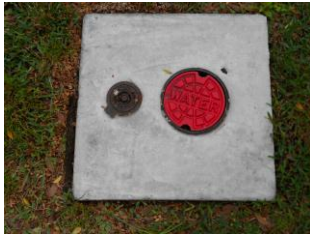
Fire Valve Box with ID
