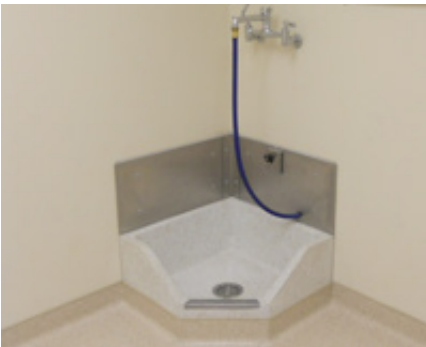
Typical Mop Sink
