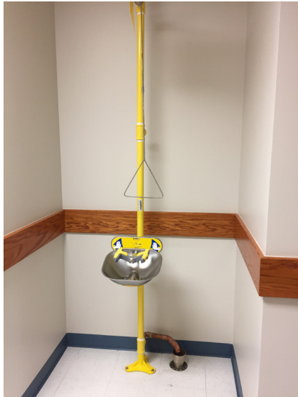
Typical Emergency Eyewash and Shower Equipment Station
