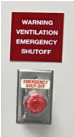
Typical Mushroom-type Resettable Button
