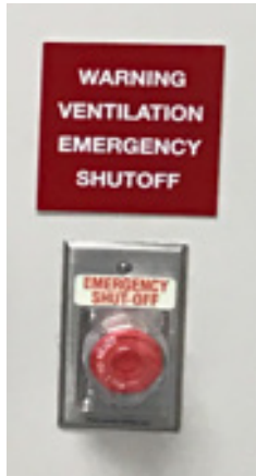
Typical Mushroom-type Resettable Button
