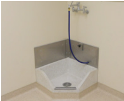
Typical Mop Sink
