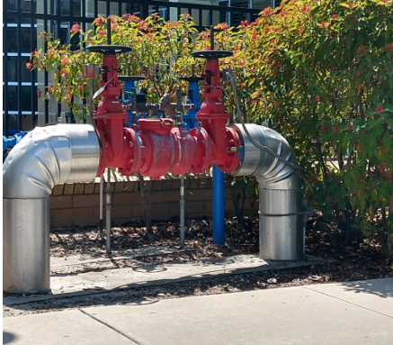
Insulation shall be jacketed finish.
