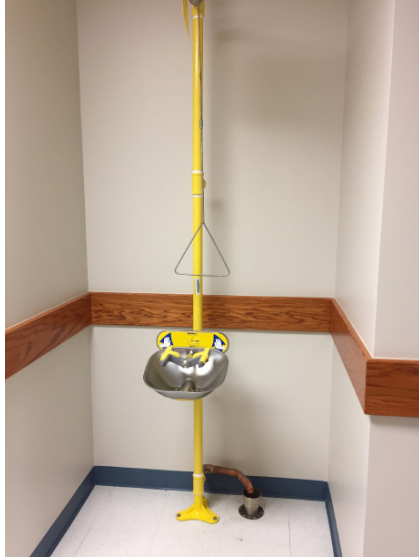
Typical Emergency Eyewash and Shower Equipment Station
