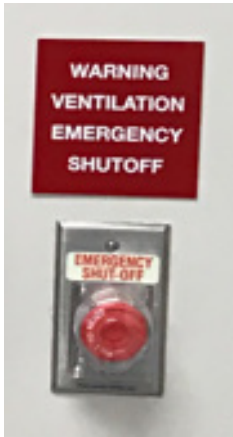
Typical Mushroom-type Resettable Button
