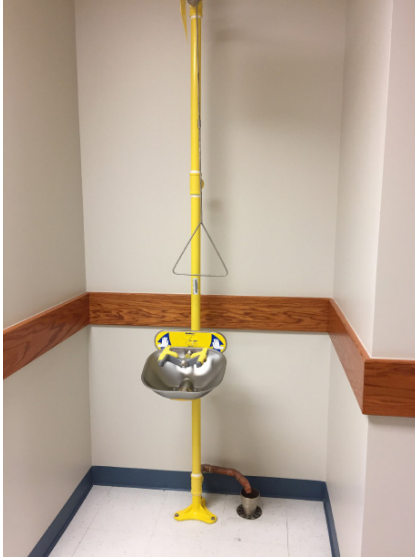
Typical Emergency Eyewash and Shower Equipment Station
