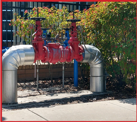
Insulation shall be jacketed finish.
