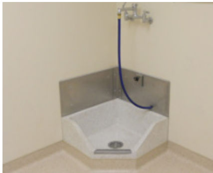
Typical Mop Sink
